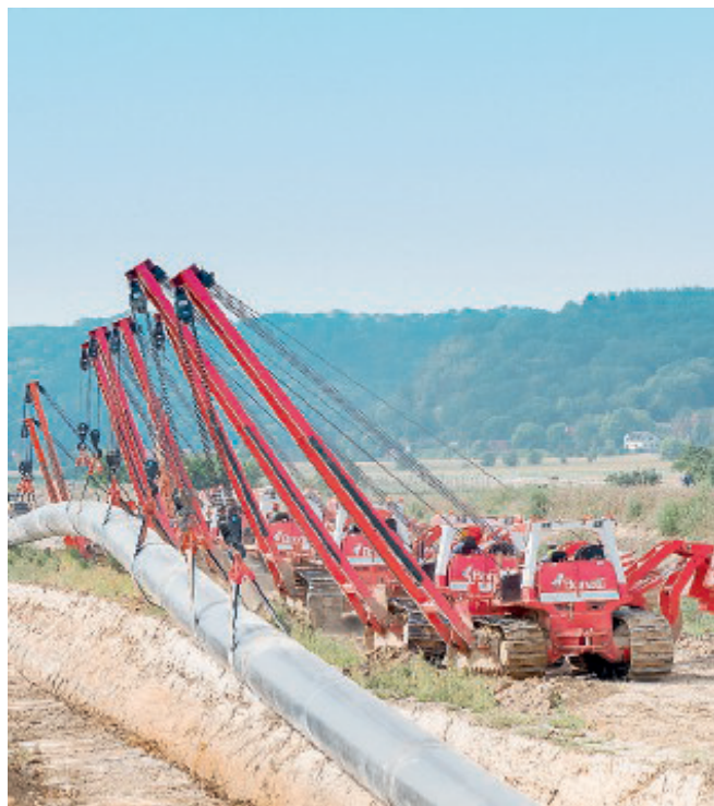
COASTAL GASLINK Bonatti in Canada gestisce 247 km.
